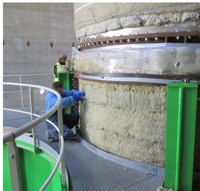
Liner fixed at the bearing platform
