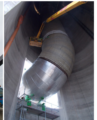
Implementation of the elbow for the connection with the horizontal flue smoke duct
