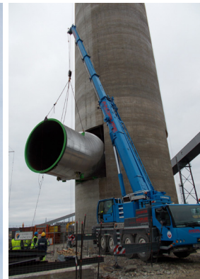
Implementation of the elbow for the connection with the horizontal flue smoke duct
