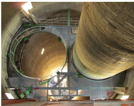
Liner fixed at the bearing platform
