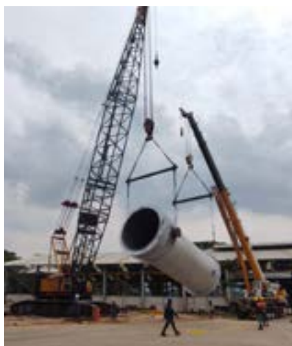
Lay down in horizontal position
