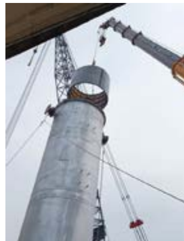
Formwork installation (1)
