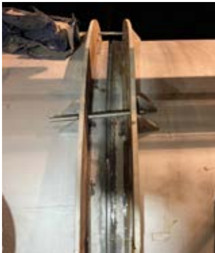
Sections aligned for welding
