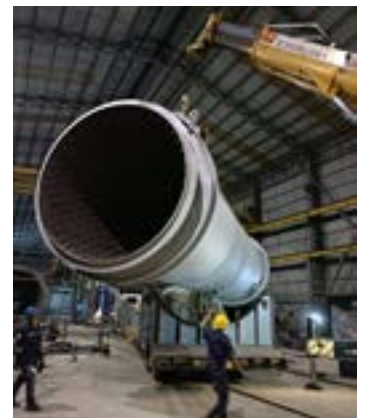
Segment relocation for lining installation
