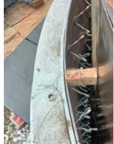
Accurate control of the lining thickness
