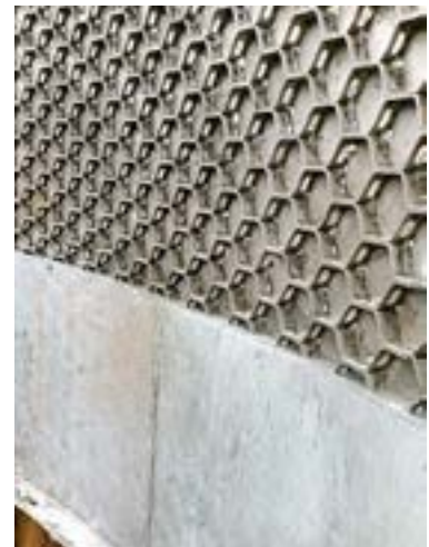
Hex-mesh for AA22 Rescobond material & Rescocast 17EC
