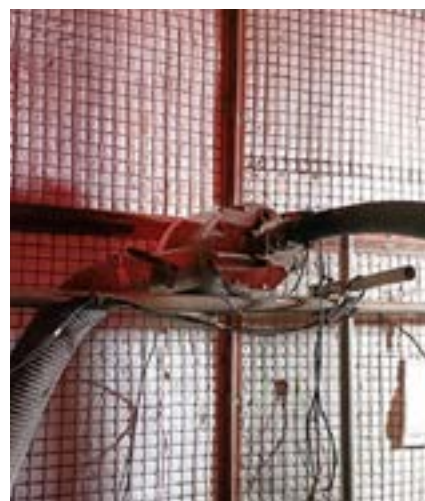
Concrete dry out (1)
