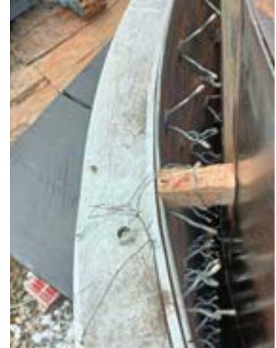
Accurate control of the lining thickness
