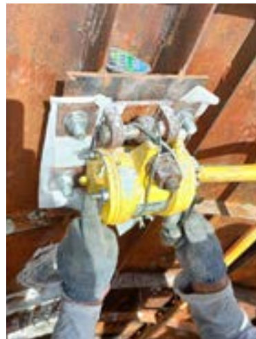
Concrete vibrator
