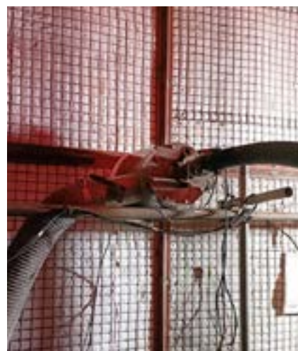
Concrete dry out (1)
