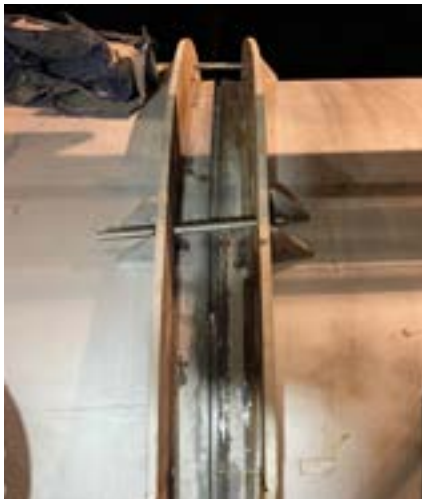
Sections aligned for welding
