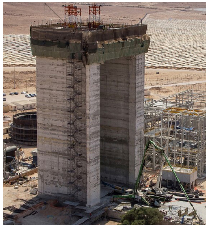
The north portion of the solar tower
