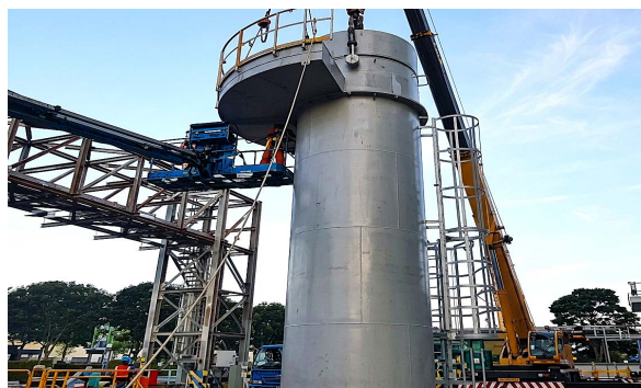
Top-mounted TMD installation
