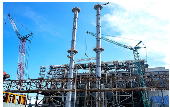
Completed stacks - view at the end of erection
