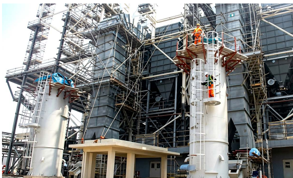
Stacks under erection - complex site constraints
