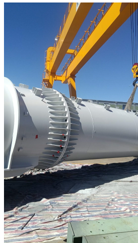
Flanges pre-assembling check
